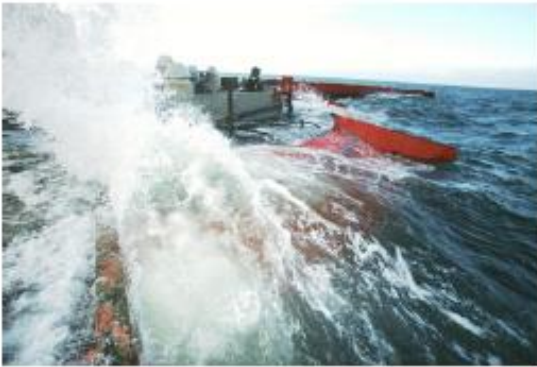
Overtopping device: Wave Dragon
