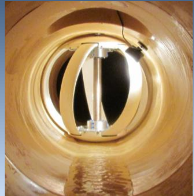
PowerPipe Installed Lemona Pump Station - Riverside, CA
