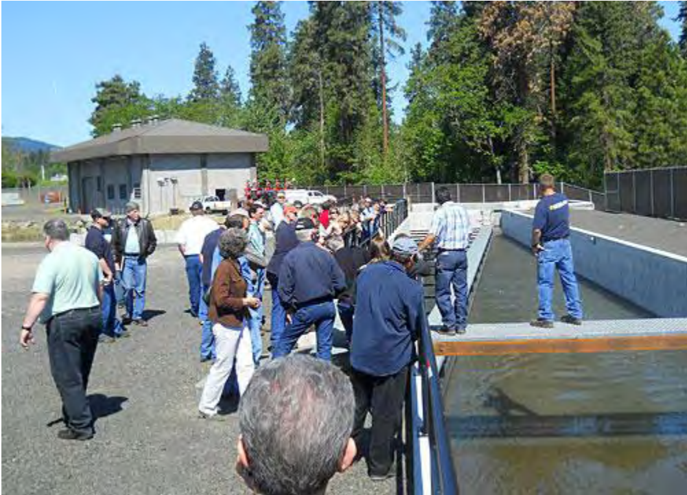
Tour of Farmers ID intake screen and powerhouse
